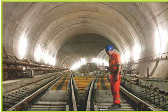
■ Tunnel Construction Project.
