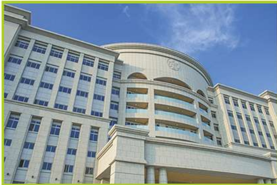
■ Natural Stone Wall Cladding Project.
