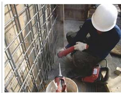
Concrete wall addition
