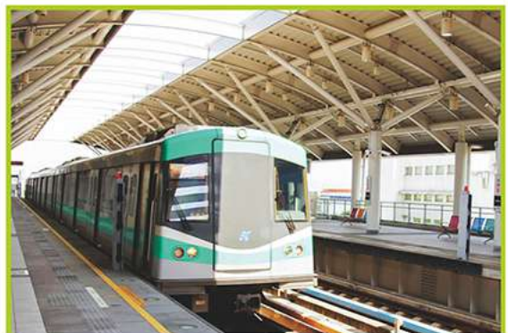
■ Kaohsiung Rapid Transit Construction Project.
